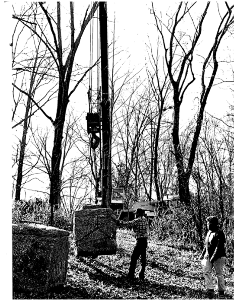
Figure 21. Installations View , Georgia, 1979, photograph from Buchanan Archives.
