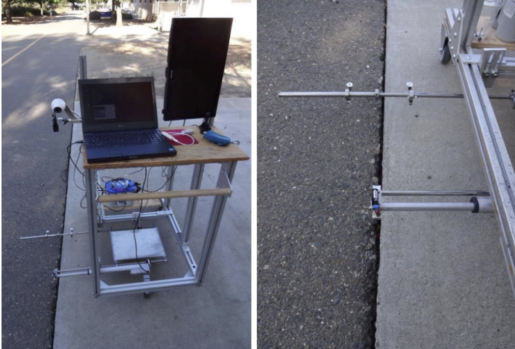
Figure 3-26 Field test: a) Integrated guidance test cart and b) Close-up actuator with the laser pointer for evaluation
