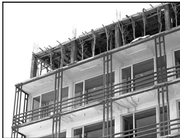
Figure 2.5. Sixth floor being added to a commercial building, central Kabul, 2003.
