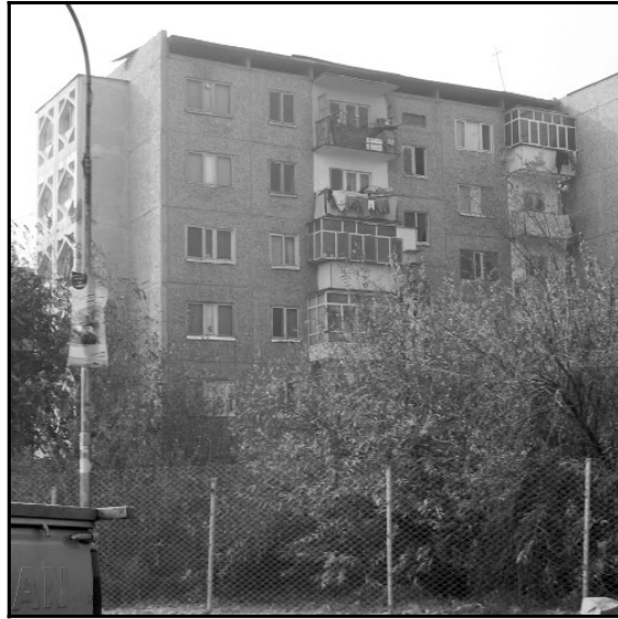
Figure 4.26. Typical six-story apartment building, Microregion 4 (author, 2007).
