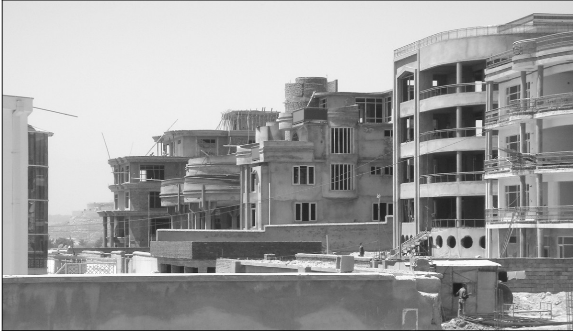
Figure 5.11. Construction in Shir Pur, April 2007 (author).
