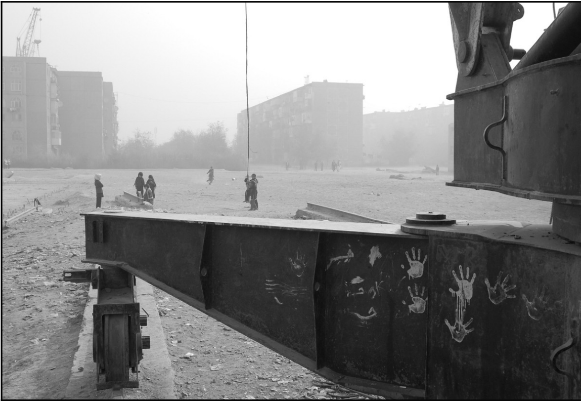
Figure 7.1. Children swinging on the hook of a crane abandoned in place in 1992. In the background is another abandoned crane and the partially-completed buildings of Micro-region 4 (author, 2007).
