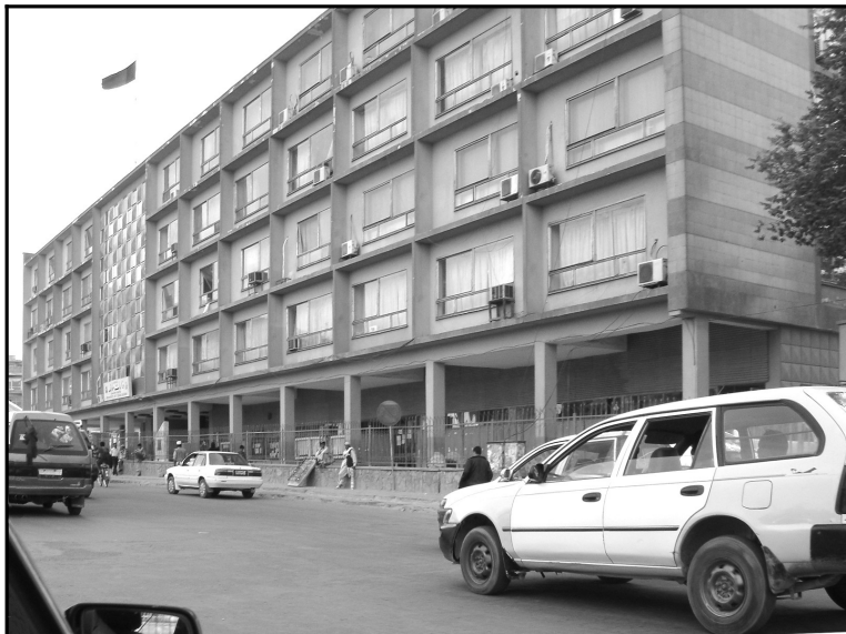
Figure 4.24. Ministry of Education, June 2006. By April of 2007 a large barrier wall was built in front of the ground-floor arcade to protect the entry area from vehicle-borne explosive attacks (author).
