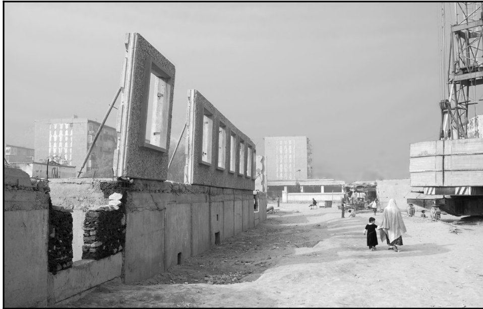
Figure 4.27. Woman and girl walk past concrete panels of incomplete building, Microregion-4. Panels were temporarily secured in place before construction was abandoned in 1992. On the lower left, the clay-brick infill wall indicates informal occupation of this unfinished building (author, 2007).
