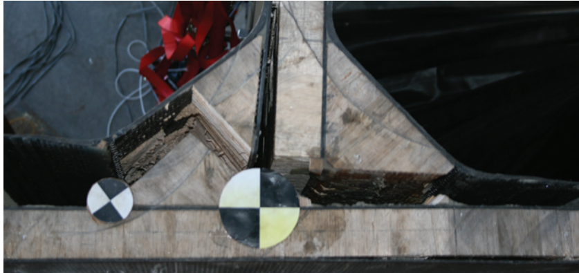
Figure 3.104: Photo of post damage in Composite Joint Test 5.
