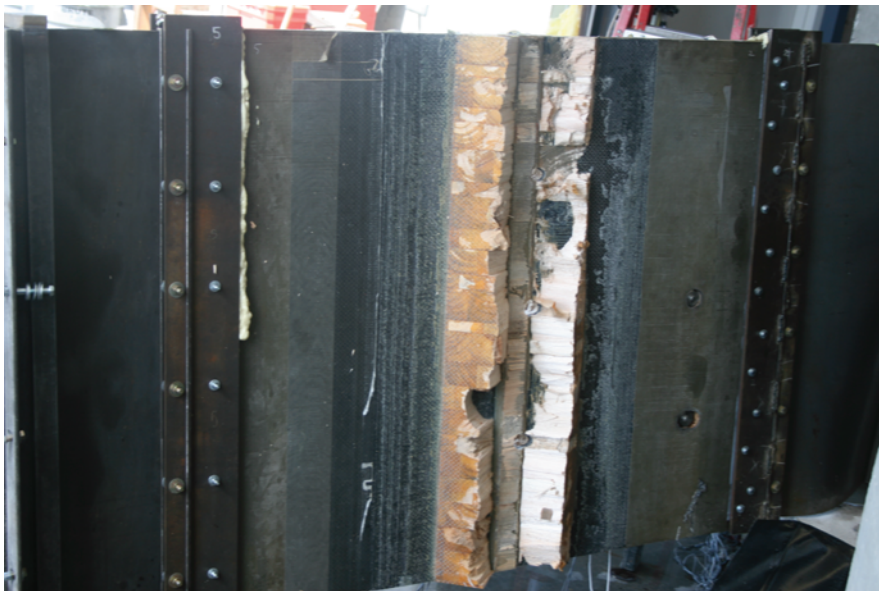
Figure 3.71: Post test photo of breached joint.
