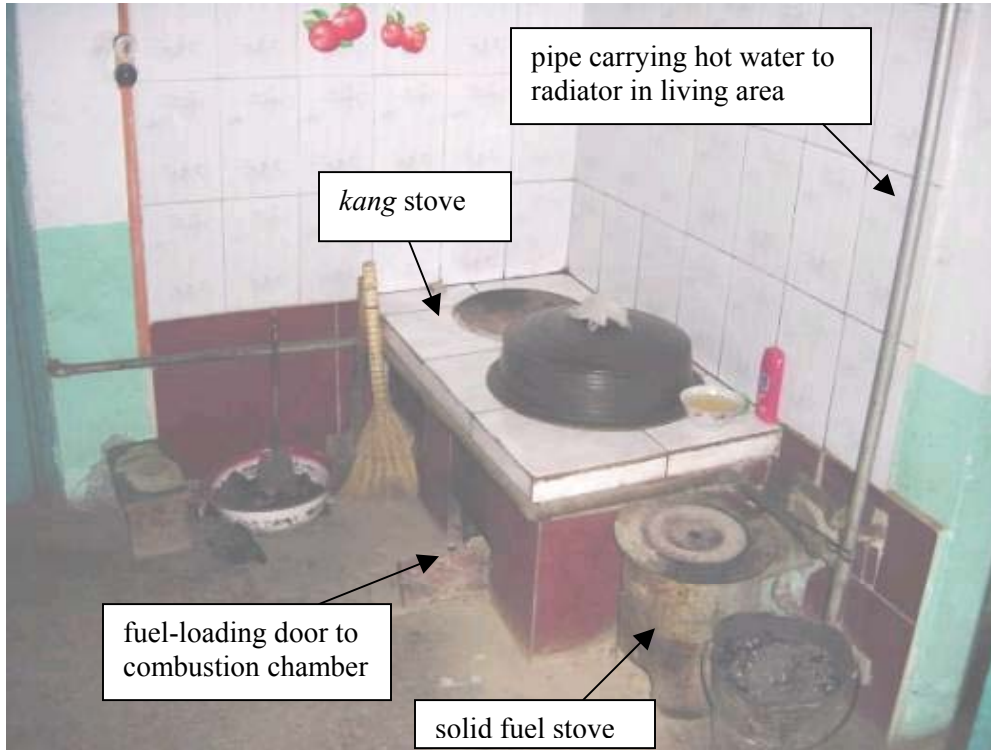
Figure 1, HECHENGLI VILLAGE KITCHEN: A Han-style kitchen showing the kang and a second solid-fuel (coal) stove for boiling tea water and fueling the radiant heating system.
