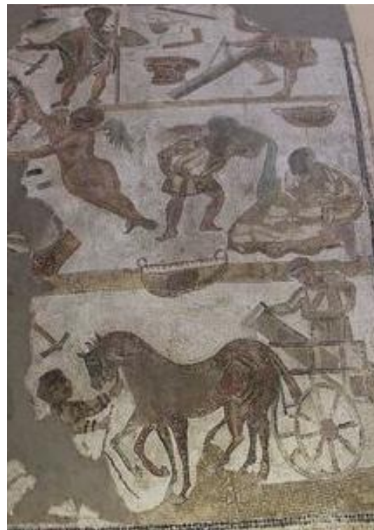
Figure 35: Mosaic of a building site. From Musedu Bardo, Tunis, Inv. A264. Photo by author.
