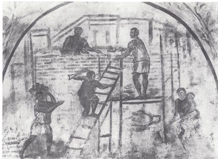
Figure 31: Masons working on a building, with bricklaying and wooden scaffolding. Wall painting from Tomb of Trebius Iustus on the Via Latina, Rome (early-4 th c. CE). British Museum, London, Inv. 299939.
