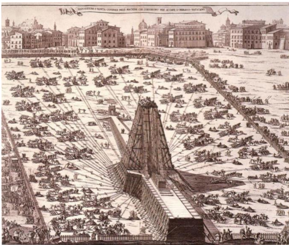
Figure 17: Sketch by Bonifacio from Fontana's manuscript depicting 330-ton Vatican obelisk being raised in 1585.
