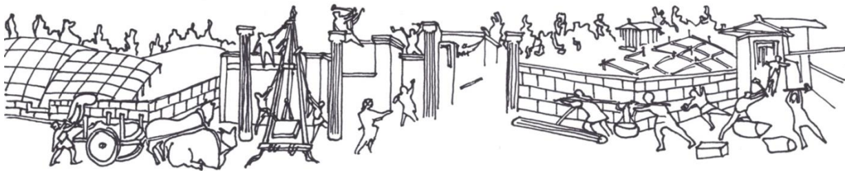
Figure 2: “Scene of a Building Site,” painting from caldarium in the Villa of San Marco at Stabiae, Archaeological Museum of Castellmare, no.282. Drawing by author.
