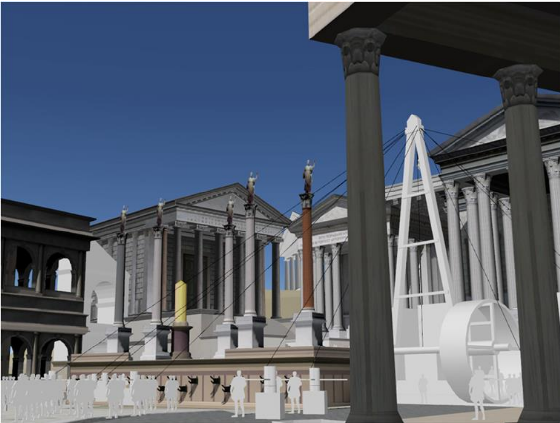
Figure 28: Rendering of a treadmill crane by the author after the Haterii Relief; in this case represented for construction in the north end of the Roman Forum. Image of Digital Roman Forum used courtesy of UCLA ETC.
