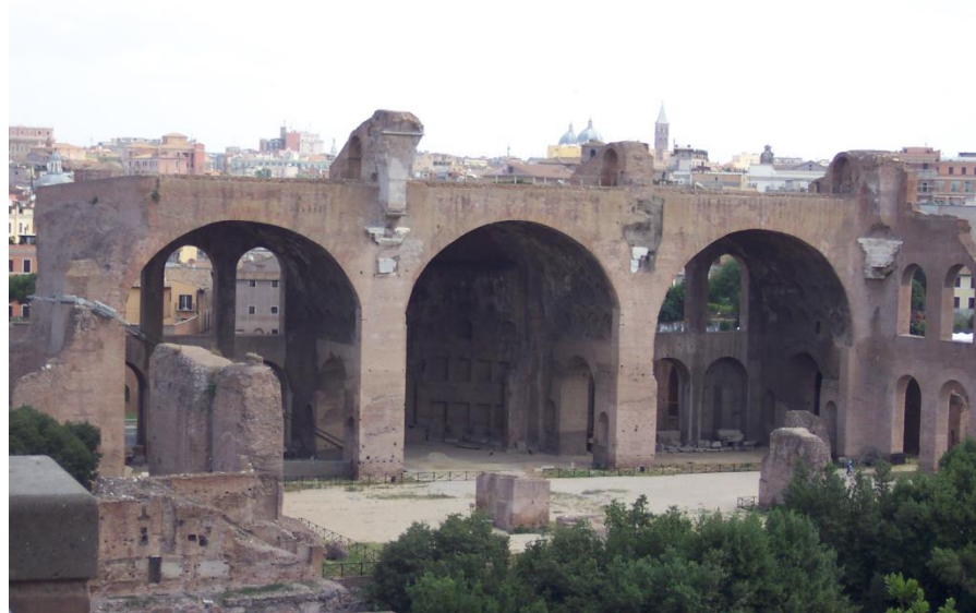
Figure 1: Current state of the Basilica of Maxentius. The northernmost aisle, or one-third, of the structure remains. This view displays only a small portion of the brick-faced concrete masonry carried out in the structure. Photo by author.
