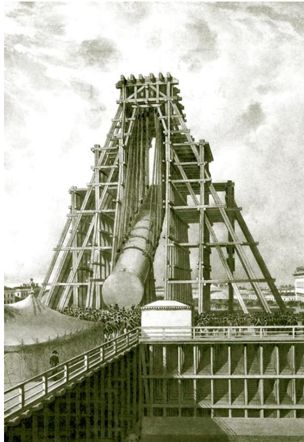
Figure 18: Sketch recording Montferrand's system for raising columns in St. Petersburg in the 1800s.
