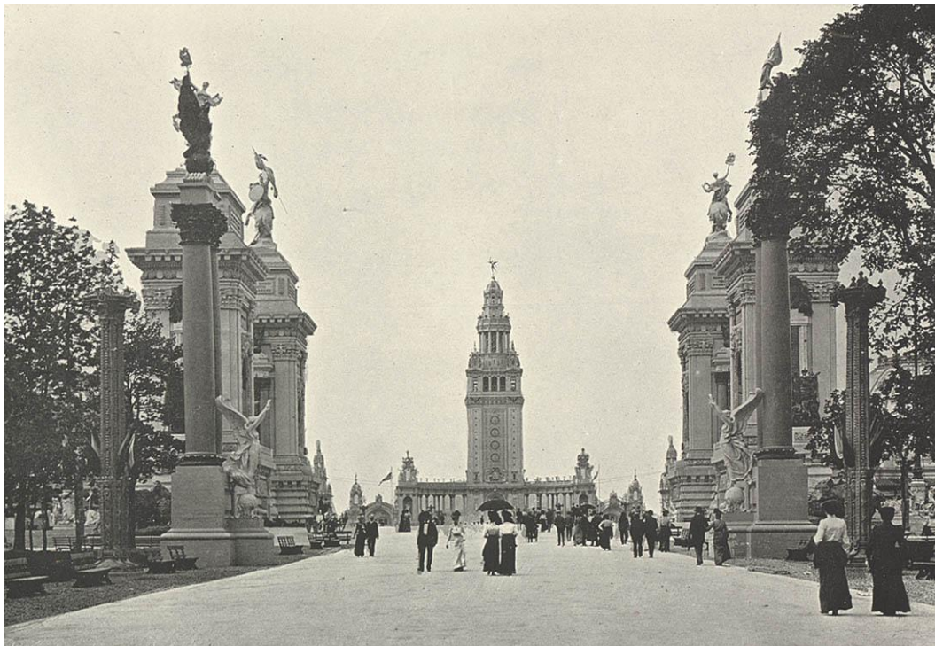
Figure 14: The Triumphal Bridge with a view of the Electric Tower at the Pan-American Exposition (1901). Photographed by C. D. Arnold from The Pan-American Exposition Illustrated by C. D. Arnold (1901). Image courtesy of the University at Buffalo Digital Collection.
