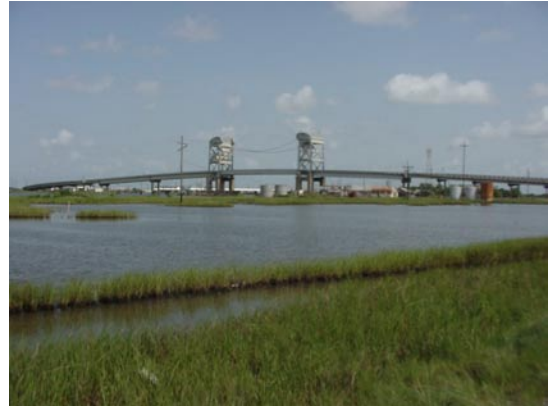
Fig. 2. Leeville Bridge – Looking North
