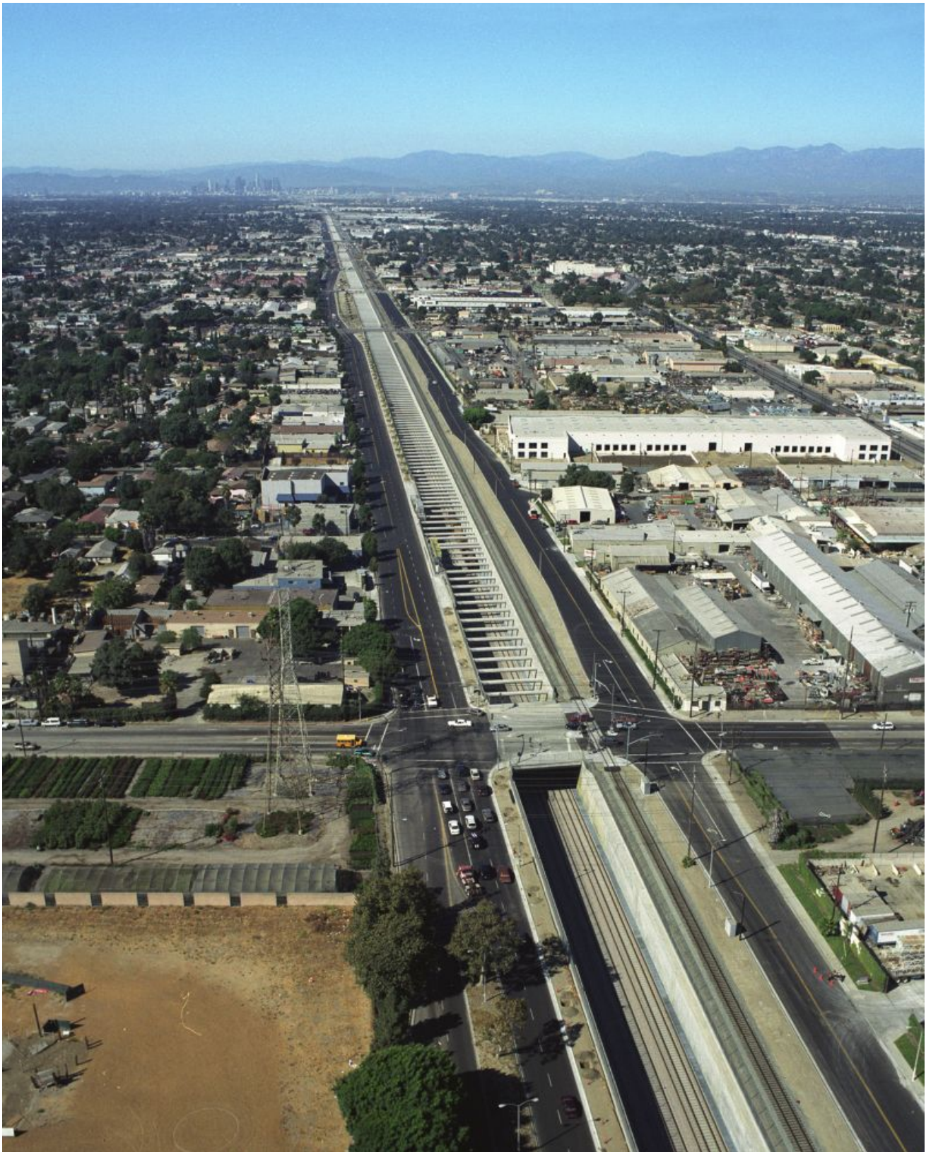
An aerial view of the trenched section of the Alameda Corridor, looking north along Alameda Street with downtown Los Angeles and its connections to the rest of the USA in the hazy distance. (Photo courtesy of ACTA.)
