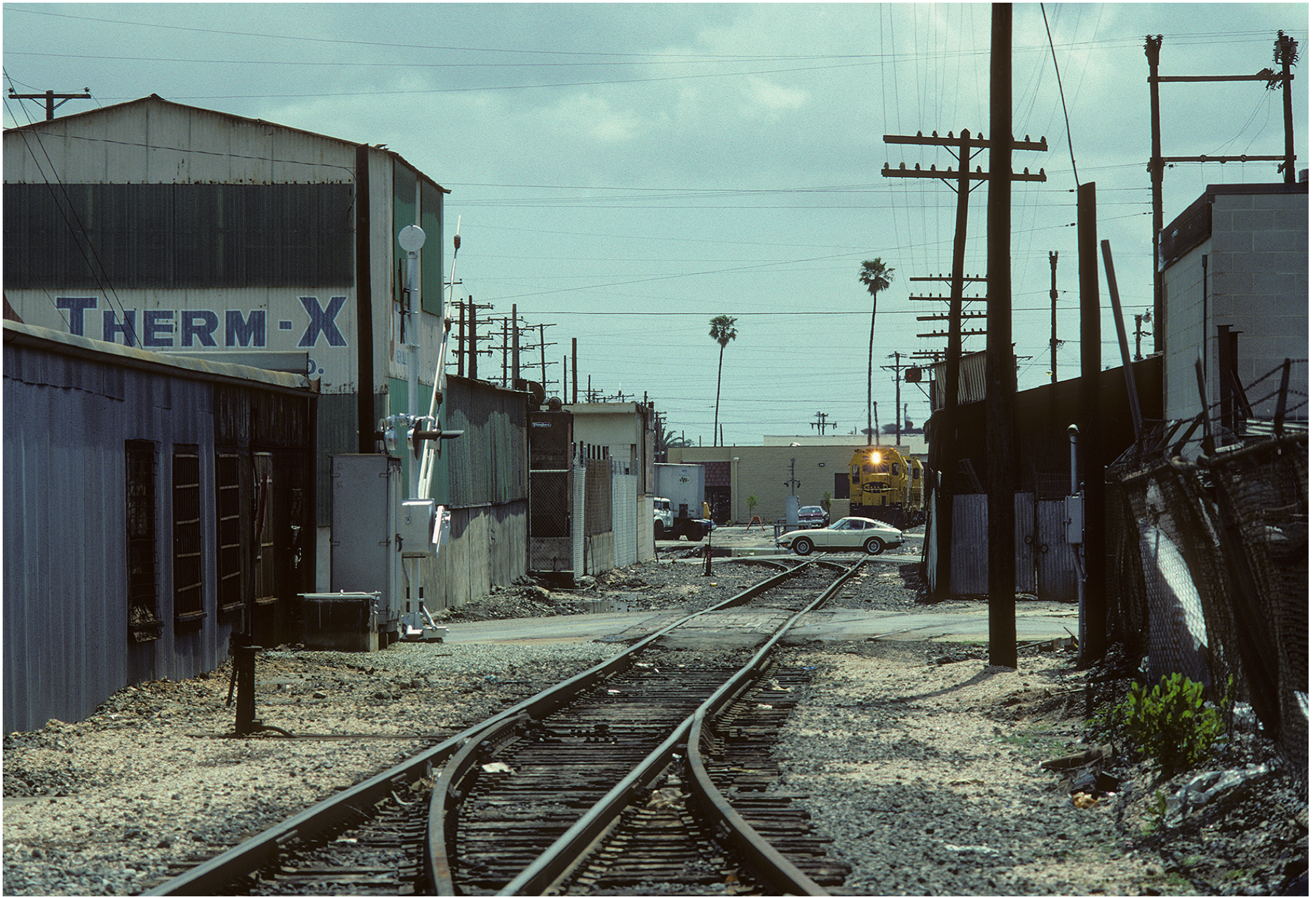
Traversing a right of way crowded by old warehouses and machine shops, a northbound Santa Fe Harbor Extra carload train creeps across the many poor-visibility crossings in Vernon near Malabar Yard, 18 April 1983.
