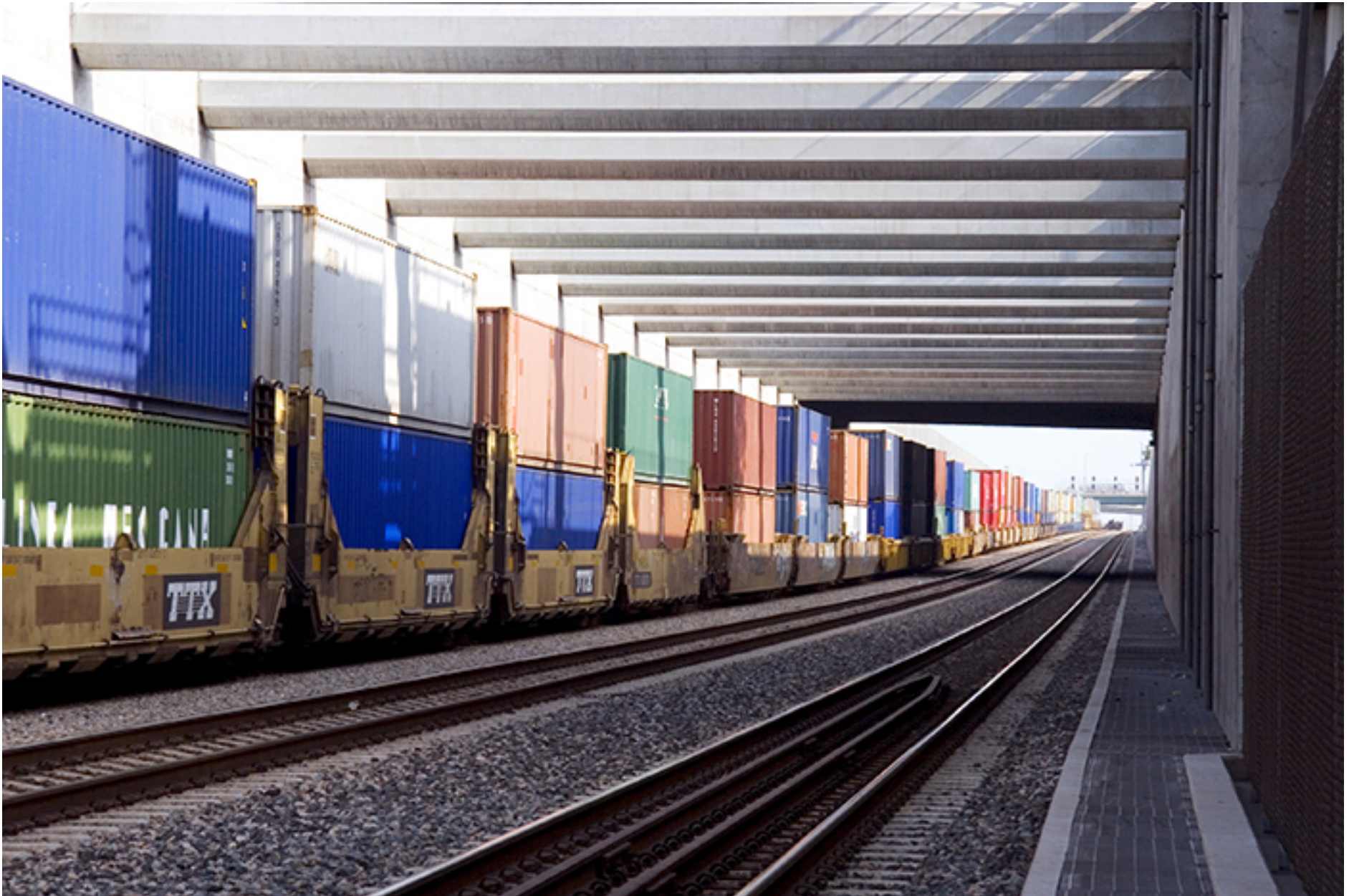
Publicity photo in the trench with some of the ocean carrier names on the container sides edited out. Although my analysis showed that two tracks would provide adequate capacity, the railroads and the Ports insisted the Corridor be built with three main tracks. This dramatically increased its cost. (Photo courtesy of ACTA.)
