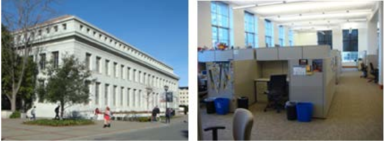
Figure 2 – Building east facade and interior cubicles
