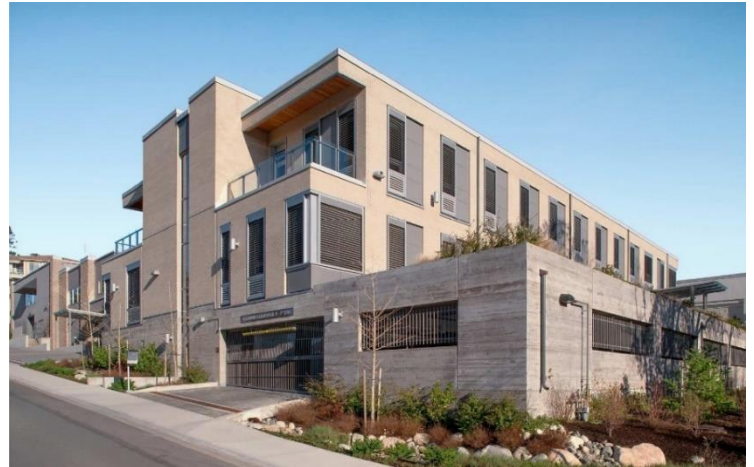
Photo: D'Ambrosio Architecture + Urbanism.
