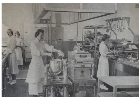
5 Nutrition lab in the new Home Economics Building, 1954
