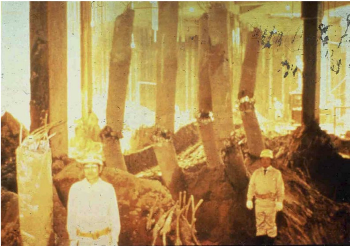
Figure 1-6. Piles supporting the NHK building sheared by lateral spreading during the 1964 Niigata earthquake (after Hamada 1991)
