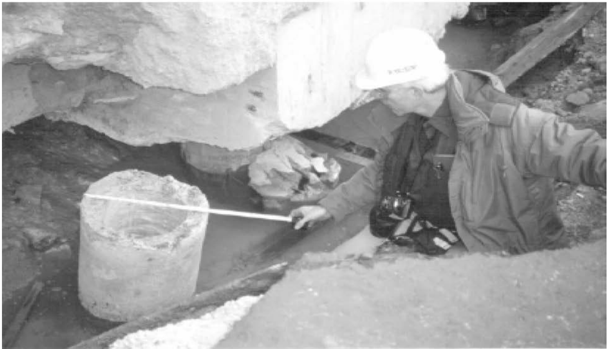
Figure 1-10. Pile shear failure during the 1995 Kobe earthquake (after Finn and Fujita 2002)
