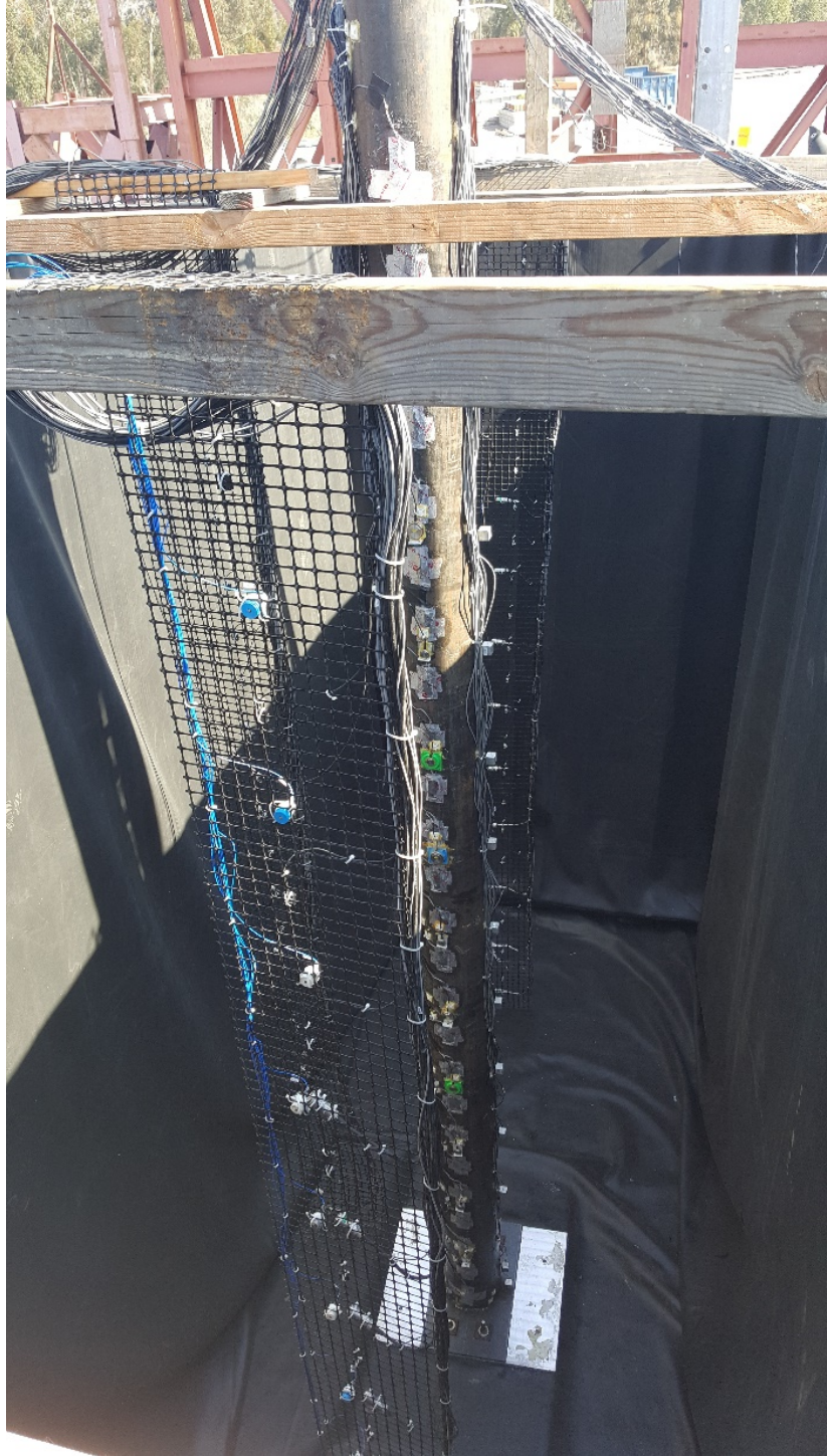
Figure 10-6. Picture of instrumented pile and free field before box filling
