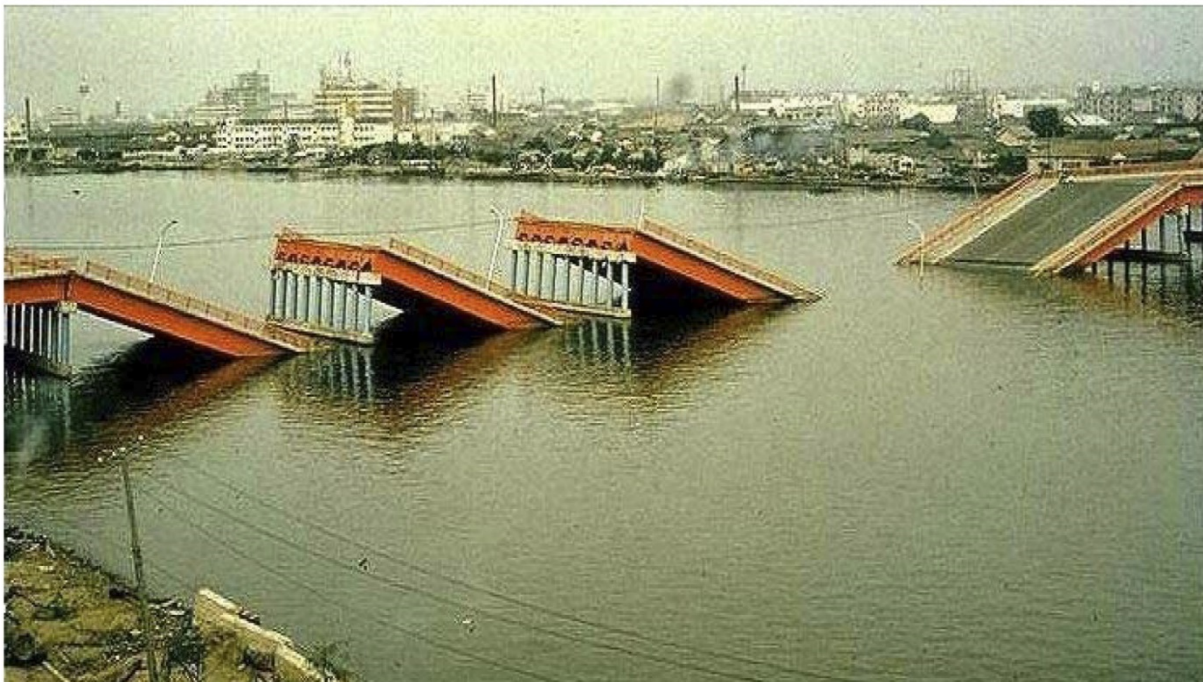
Figure 1-4. Collapse of the Showa Bridge due to unseating resulting from large lateral displacement of its pile foundations during lateral spreading induced by the 1964 Niigata earthquake (after NISEE)
