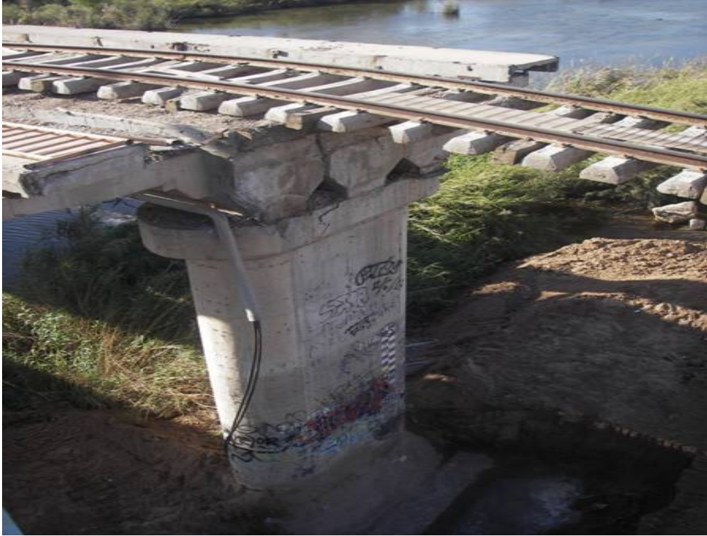
Figure 1-17. Unseated pier caused by lateral spreading, Photo by Scott Brandenburg (GEER Association Baja California 2010b)
