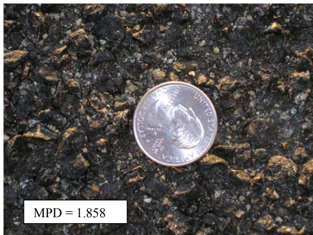
#1 5/16" PME seal coat (PM 4.5-4.7)
