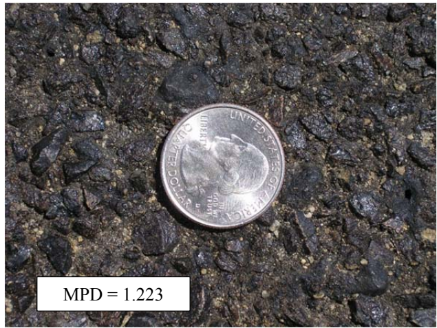
#6 1/4" PME seal coat - double chip seal (PM 10.0-9.8)
