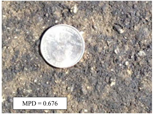
#8 Slurry seal (PM 9.4-9.6)
