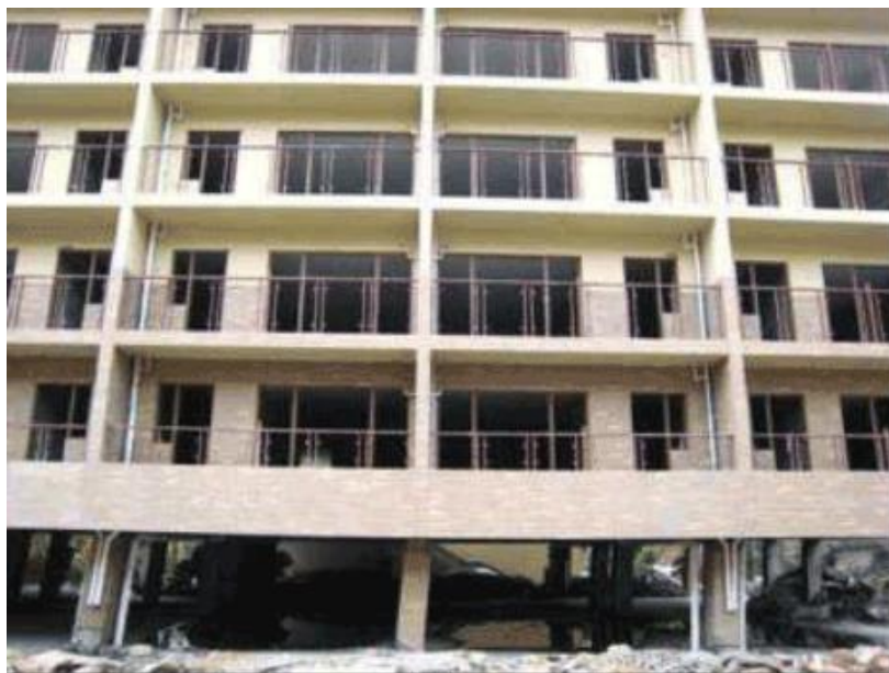
Fig 1.3: A six storeyed building with soft-storeyed ground floor at Dujiangyan in 2008 China earthquake
