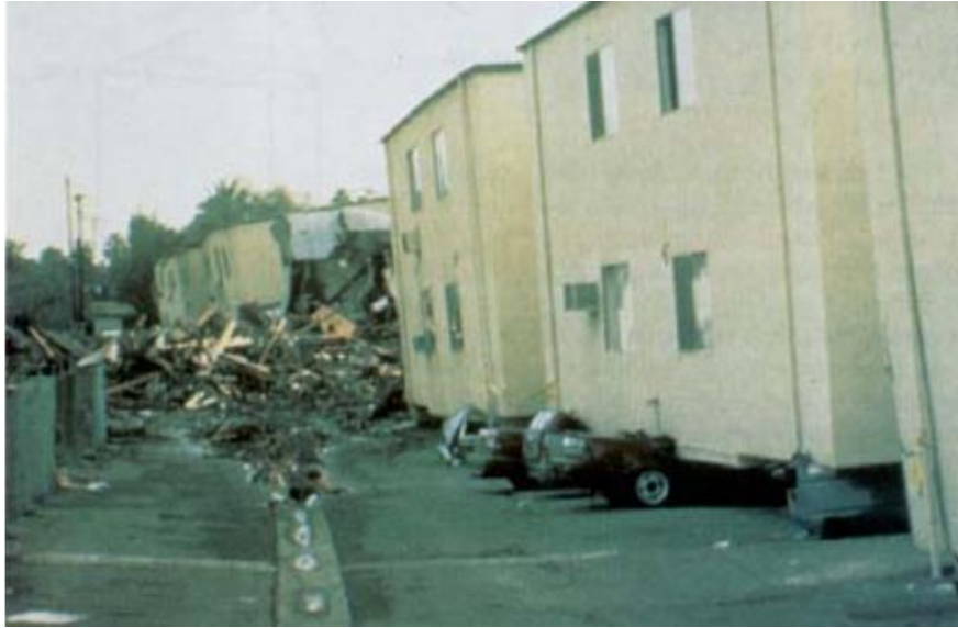
Fig 1.4: Total collapse of soft storeyed open garage at the ground floor of the apartment building in Northridge earthquake
