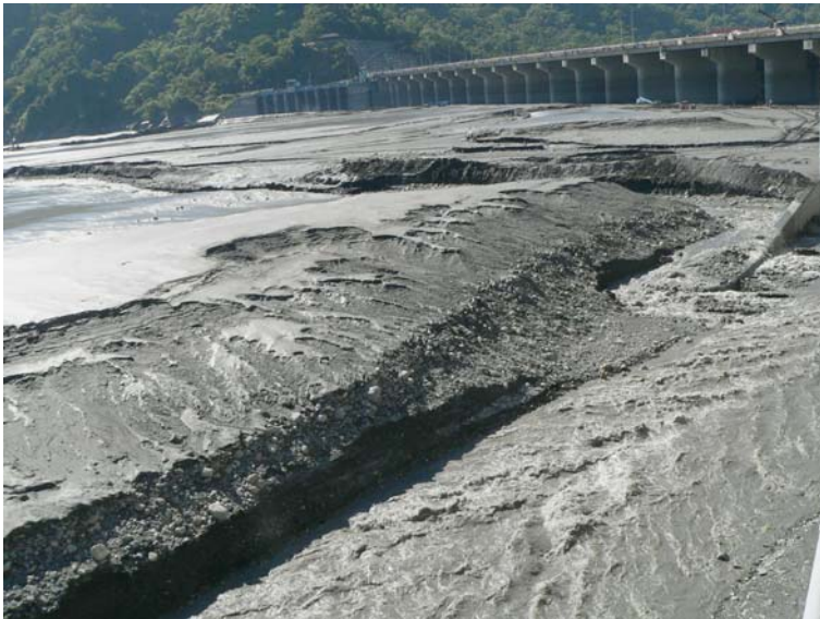
Fig. 2 Siltation upstream of the weir of the Jiji (Chi-chi) reservoir (Taiwan) on the Zhoushui River, on November 11, 2008. The reservoir sediments are regularly dredged for construction materials
