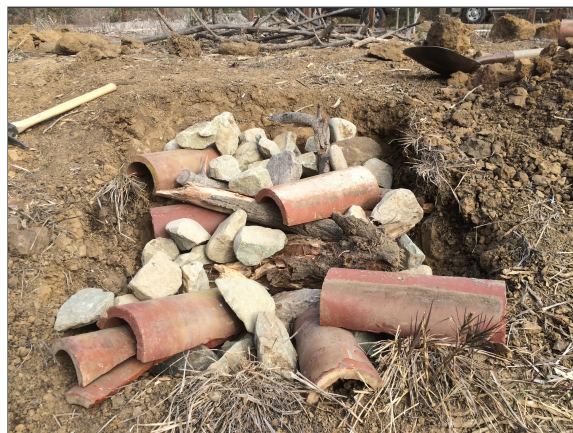
Hibernaculum construction: pipe supplies water to underground reservoir, and "urbanite" material provides many layers and spaces.
