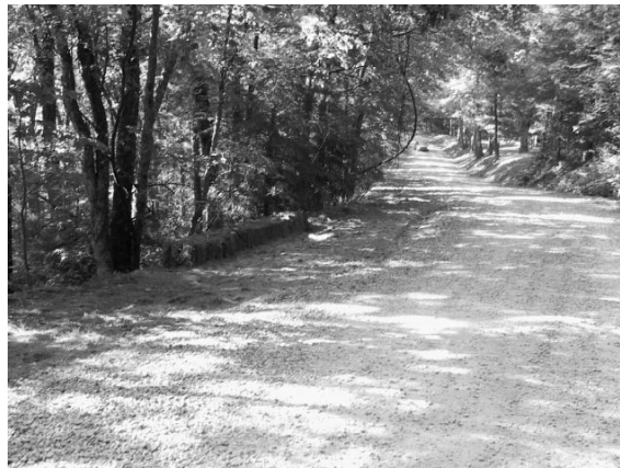
Fig. 3. A re-constructed forest road illustrating best management practices.
