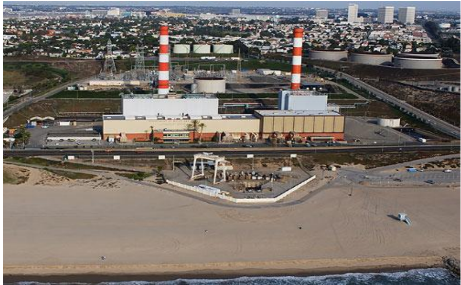
Figure 4. The Scattergood power plant in El Segundo, CA, owned by the LADWP. (California Coastal Records Project)
