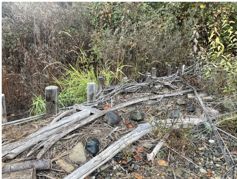
Figure 2. Example of vertical reinforcement posts in a BDA installed by Scott River Watershed Council. 11/4/23, Etna, CA.
