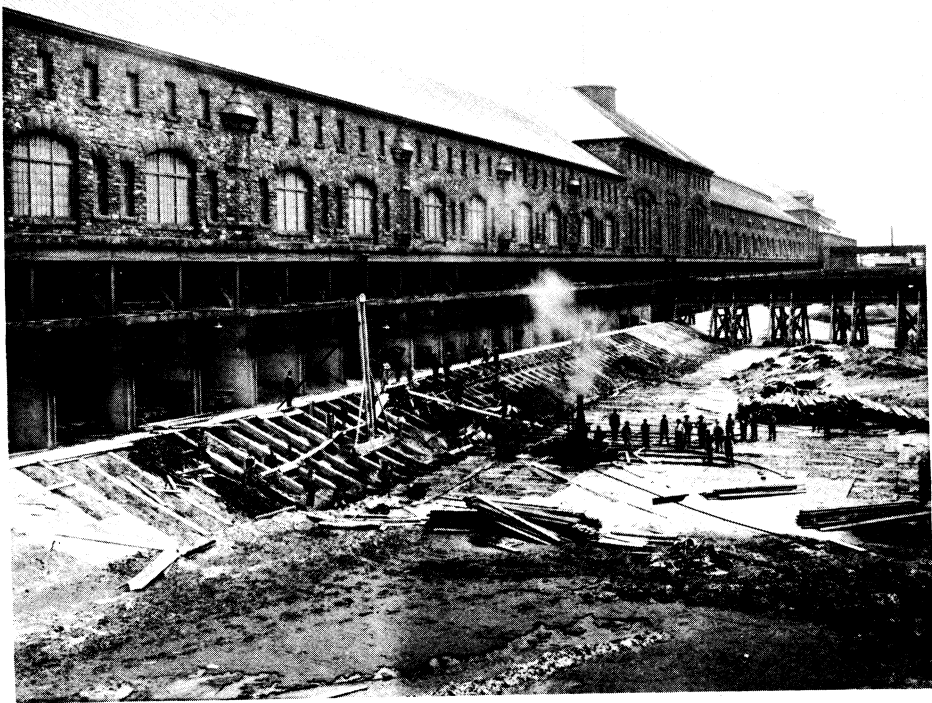
1910 view of the Michigan Lake Superior Power Company's powerhouse in Sault Ste. Marie, Michigan, as it undergoes foundation repair.
