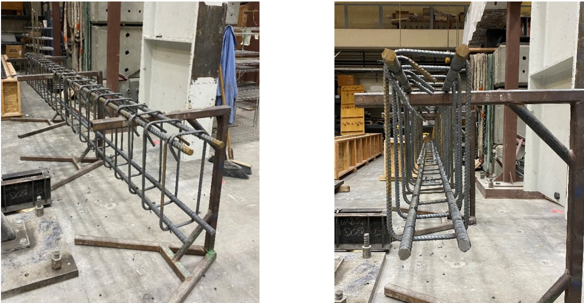
Figure 3-17: Rebar cage assembly of large beam specimens
