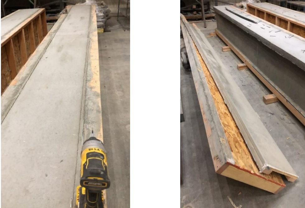
Figure 3-19: Formwork removal of large beams
