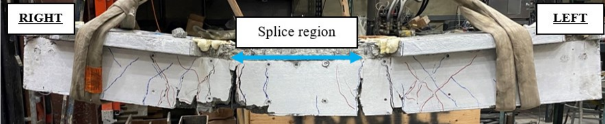
Figure 4-11: SB-S2-20 at the end of the test
