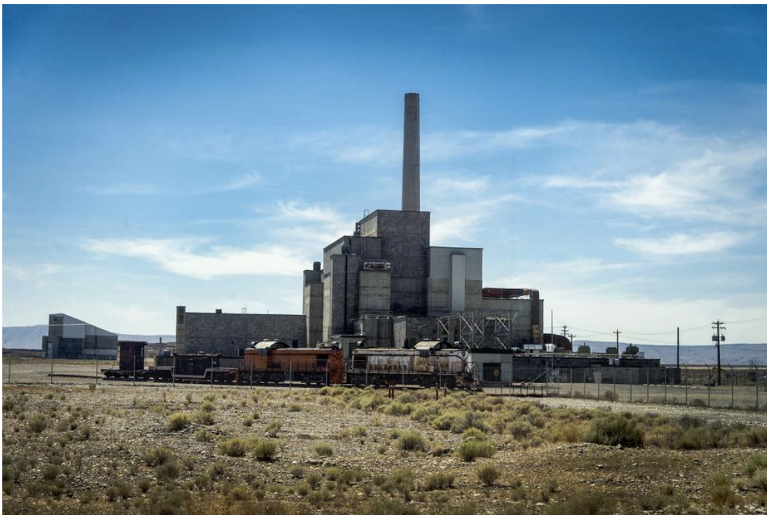
6. Hanford’s B Reactor (Mulvany 2014).
