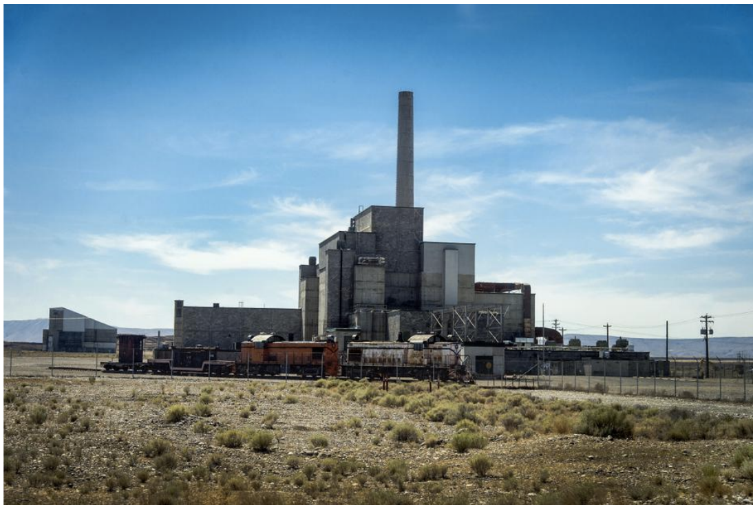
6. Hanford’s B Reactor (Mulvany 2014).
