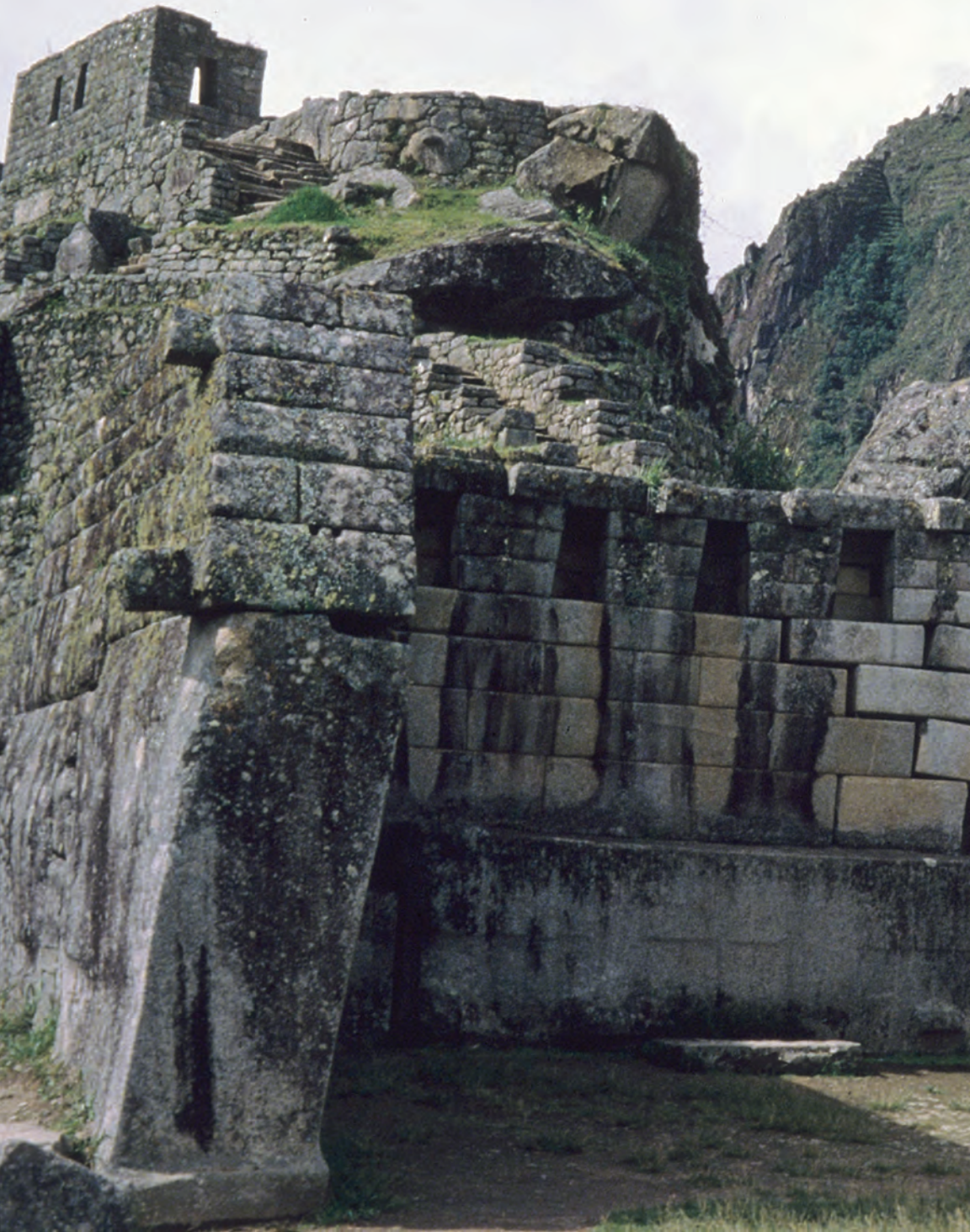
Figure 3.7. This structure was named the Principal Temple by Hiram Bingham. Sand was found to cover the floor of the temple.
