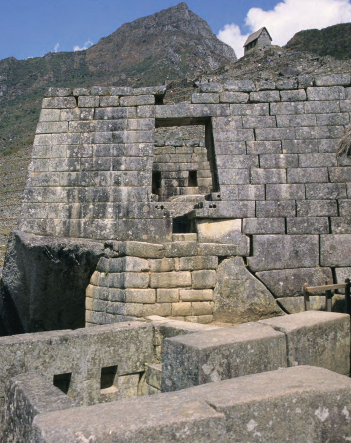
Figure 3.28 (left). Water was routed from the lower right in this view north toward Machu Picchu from the northern slope of the mountain for which it is named.
