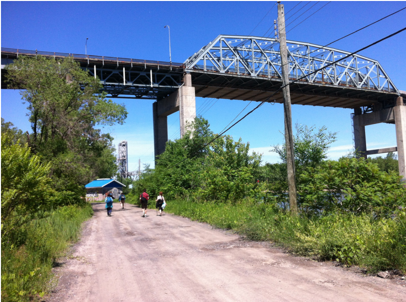
Service Road between Ville de Ste-catherine and Kahnawa:ké, with Mercier Bridge.
