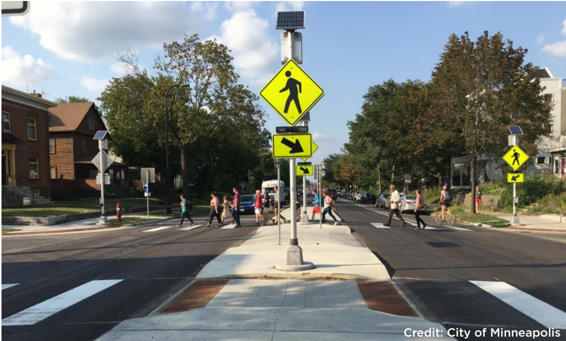
Pedestrian safety islands with curb ramps
