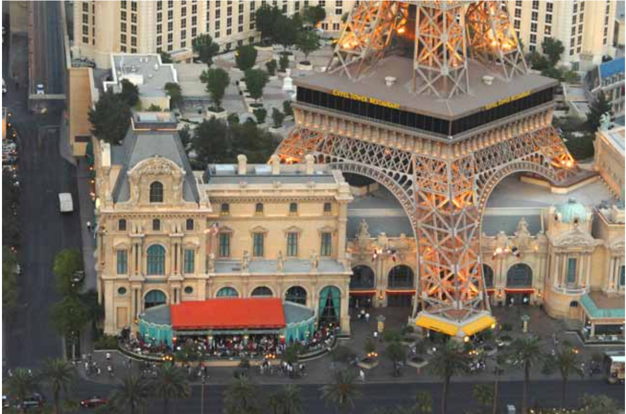
Image 51) In a departure from the original, the half-size replica of the Eiffel Tower stood partly outside on the Strip, partly inside the casino, at Paris Las Vegas, to make it visible all the time. [41]
