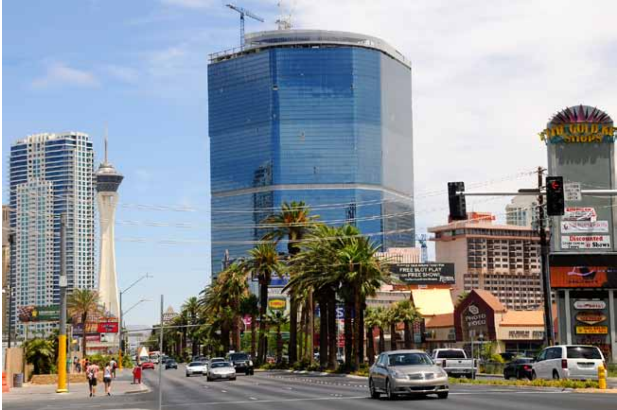
Image 26) As a result of the condominium boom, the number of high-rises on the Las Vegas Strip had increased. In the center, the 63-story Fontainebleau is under construction. Sky Las Vegas, a 45-floor condominium tower, can be seen on the left. [22]
