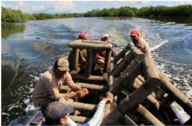
Figures 6 and 7. The deployment of artificial reefs in the Bay of Jiquilisco. This type of artificial reef is called “cubo,” meaning cube. These reefs were deployed with help from CENDEPESCA and USAID in 2015, and may be similar to the reefs used by the fishing cooperatives based near Puerto Parada. Photos by David Alfaro (Lopez 2015).
