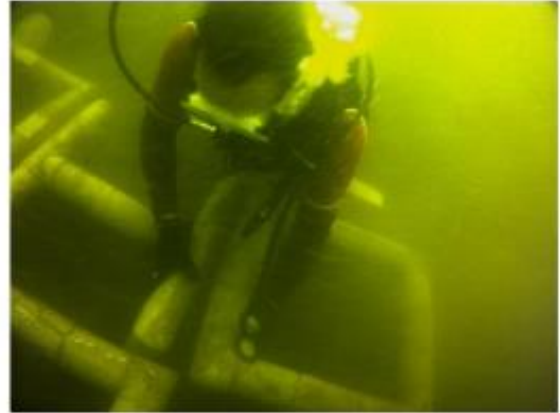
Figures 6 and 7. The deployment of artificial reefs in the Bay of Jiquilisco. This type of artificial reef is called “cubo,” meaning cube. These reefs were deployed with help from CENDEPESCA and USAID in 2015, and may be similar to the reefs used by the fishing cooperatives based near Puerto Parada. Photos by David Alfaro (Lopez 2015).
