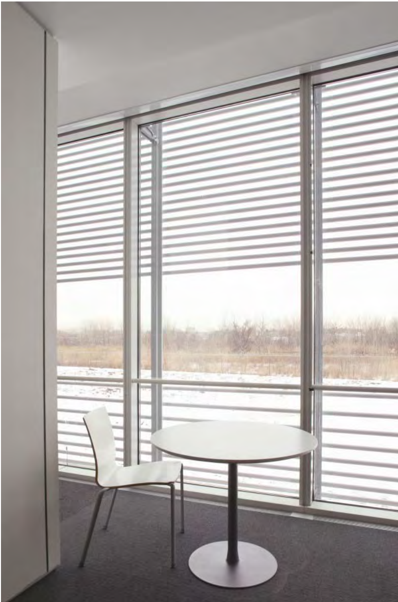
Figure 5. The view section of the window wall is the open portion between the upper and lower exterior shading elements (photo from the daylighting mockup at College Point, New York). Copyright: LBNL.
