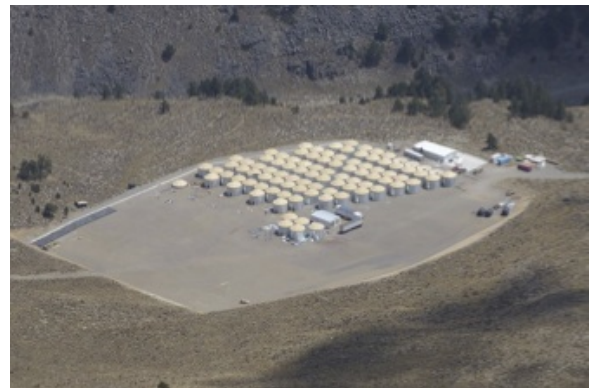
Figure 2: Aerial view of the HAWC array taken in April 2013.
