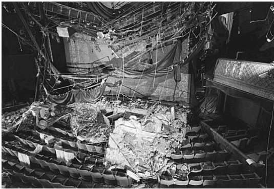
Fig 1. The Geary, following the 1989 Loma Prieta Earthquake
