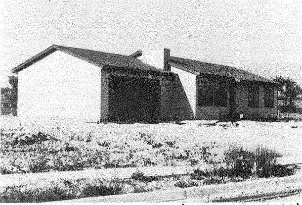
Figure 13. South facade of Prowswood/HUD house incorporating return-air windows and sun tempering system.
