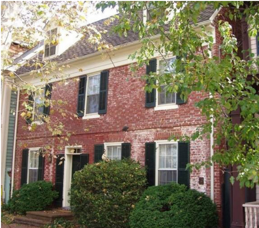
Figure 1 Patrick Henry House, 103 N Queen Street, Chestertown, Maryland, 1730-35.
