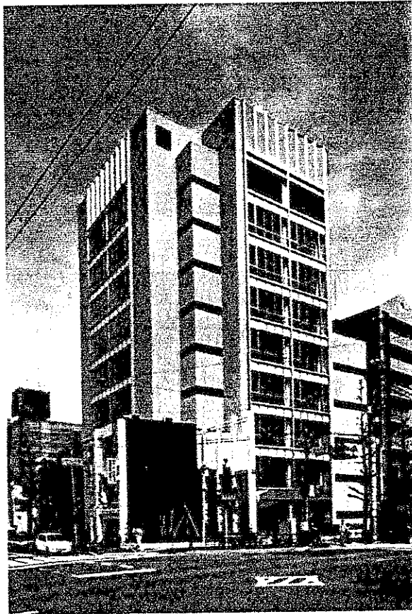
Figure 3.3 Exterior view of the KKE building (courtesy of KKE)
