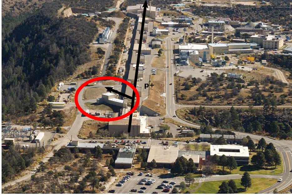
Figure 2.13: Aerial photograph of the LANSCE beamline. Proton injectors are seen in the foreground building near the arrow's tail. The IPF beamline and operations facility is seen to the left of the main LANSCE beamline, circled in red. The target box seen in Figure 2.1 is lowered into the beamline here, via a hot cell.
