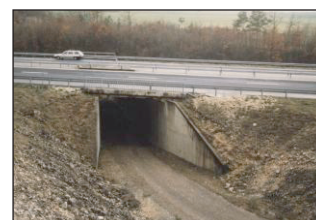
Fig. 3. 2 nd generation of fauna passages. Underpass at the A5.
