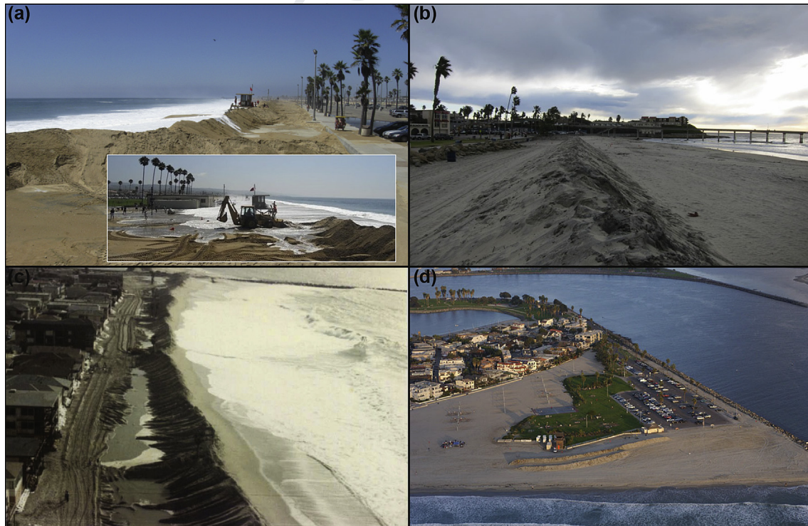
Fig. 1. Examples of anthropogenic beach berms at (a) Balboa Beach August, 2011, inset photo shows end flow around the berm edge (b) Ocean Beach December, 2011 (photo used with permission, George Fatell) (c) Seal Beach, 1983 (McMahon, 2009) and (d) Mission Beach, October 2006, photo used with permission, ©2002–2013 Kenneth and Gabrielle Adelman, California Coastal Records Project www.Californiacoastline.org .
