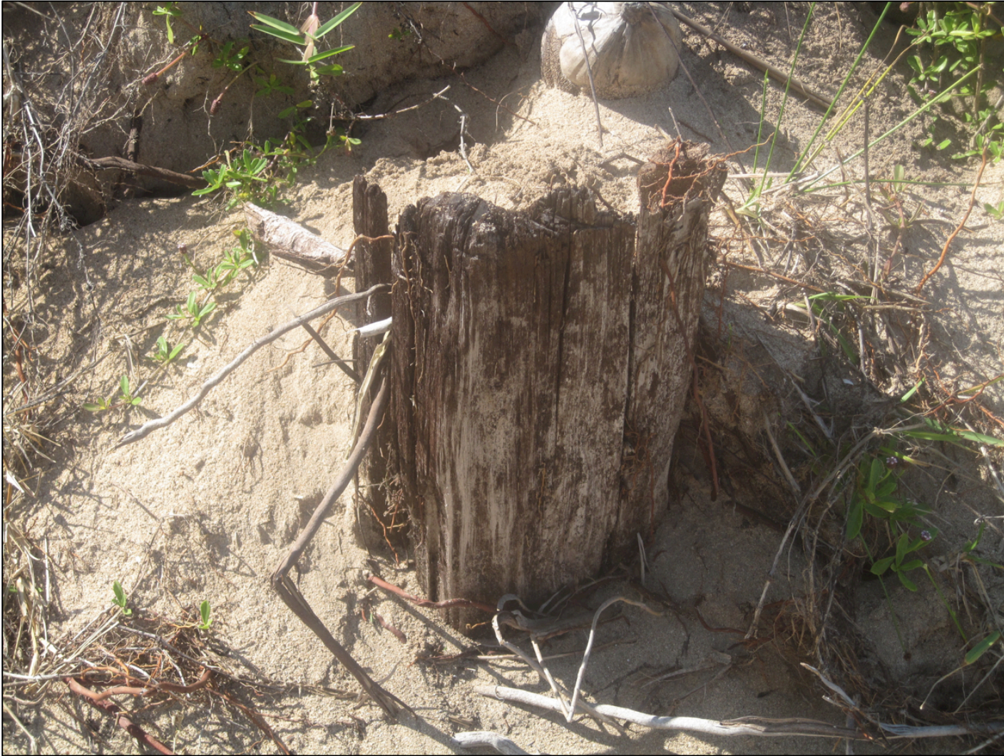
Figure 13: Wood Post from Historic Foundation
