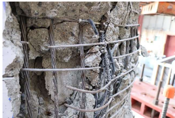
Fracture of wire spiral at 2.5% drift
