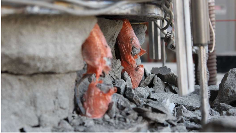
Figure 9.10: Picture showing rebar bending and fracture in sacrificial region of Specimen 1 after the test
