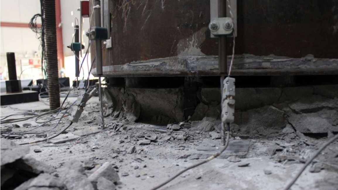
Figure 9.43: Picture of south side of Specimen 2 after first cycle at 5.01% drift ratio
