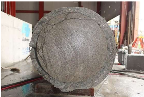
Section right above core bars
