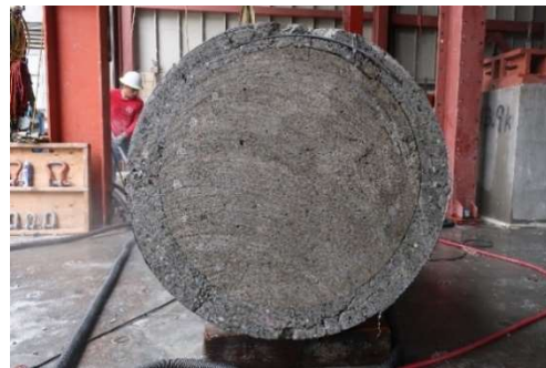
Section right above pile cap soffit
