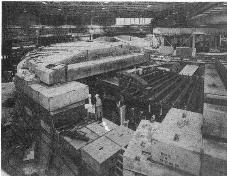
Fig. 6.85. View of Bevatron shielding under construction.
