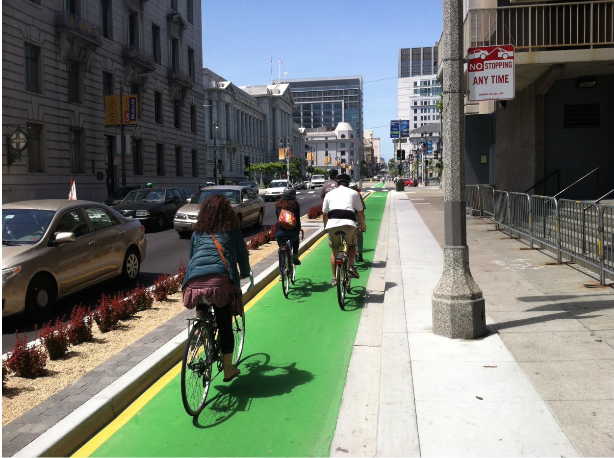
Figure 6. An example of a physically separated bicycle lane in San Francisco
