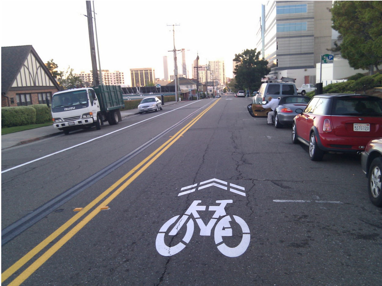
Figure 1. A bicycle route marked by a sharrow (photo credit: Eric Fischer)
