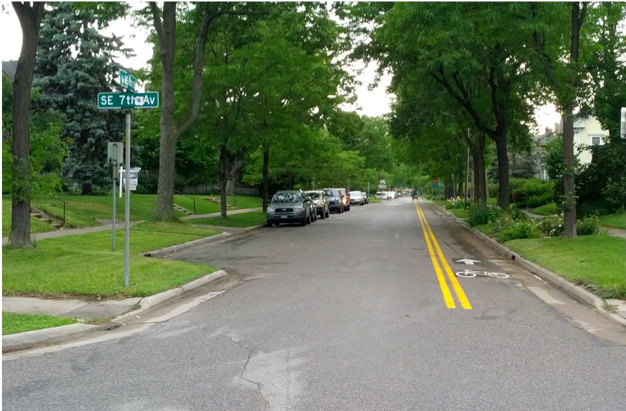
Figure 5. An example of a contraflow bicycle lane (photo credit: Eric Fischer)
