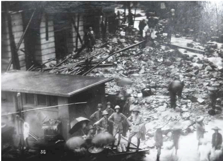
Figure 4.11. A scene of a house collapse in Victoria. (Source: The National Archives of the U.K.: Public Records Office, London).
