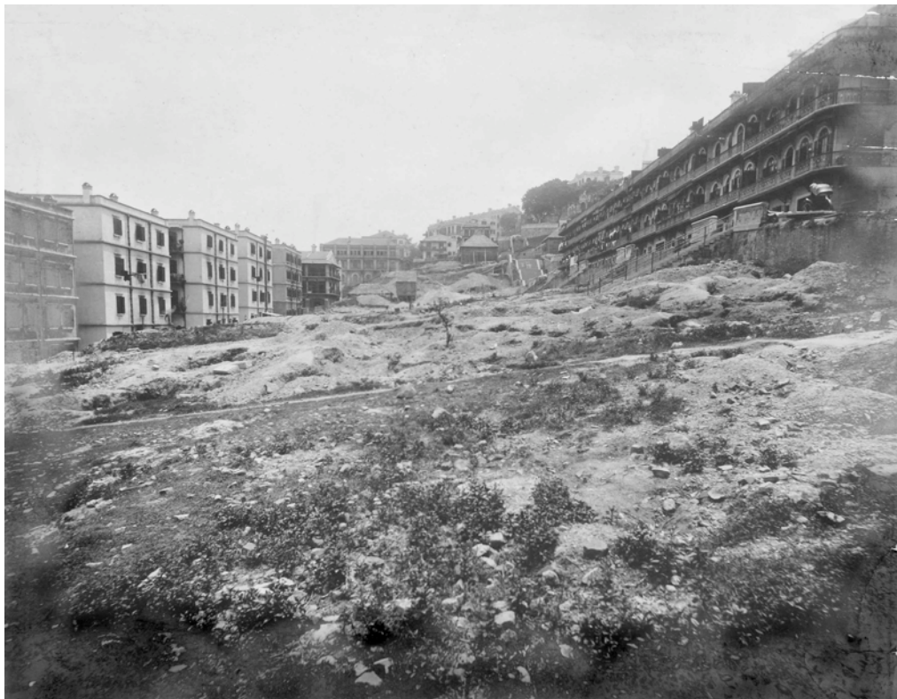
Figure. 3.12 and 3.13. Two views of Taipingshan after the demolition, 1895. (Source: The National Archives of the U.K.: Public Records Office, London).
