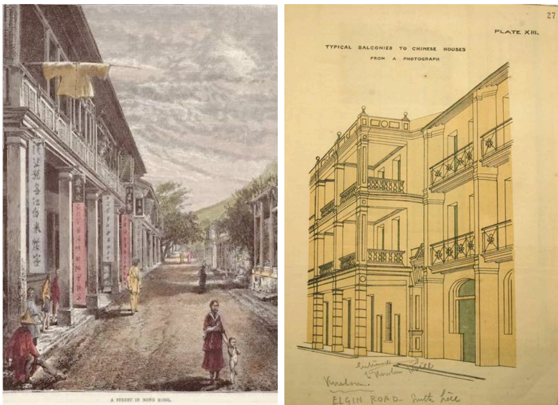
Figure 2.7 & 2.8. Two drawings showing the verandahs of tong lau . (Source: The National Archives of the U.K.: Public Records Office, London).
