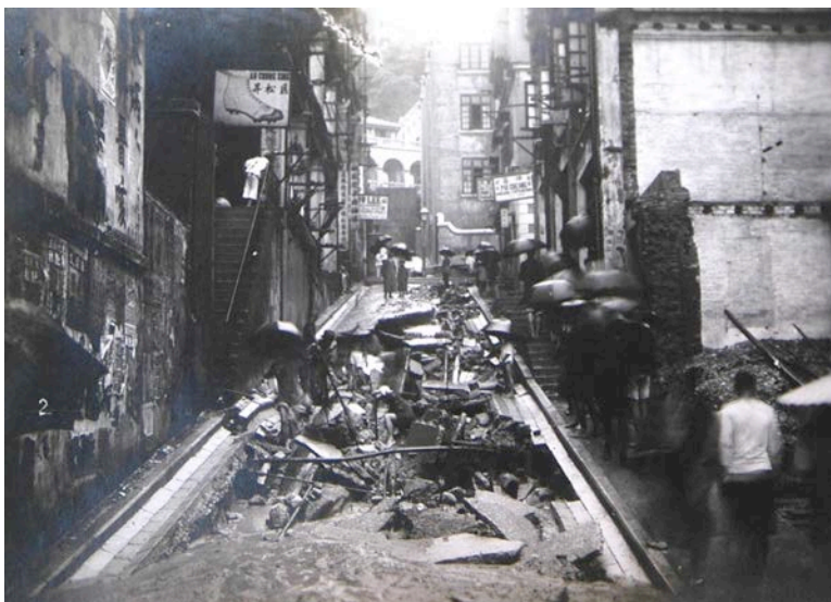
Figure 4.12. Road damage after a typhoon in the Central District. Government contractors had been criticized for using inexpensive soft stone in place of more enduring materials for the construction of roads, leading to their quick deterioration and many accidents. (Source: The National Archives of the U.K.: Public Records Office, London).
