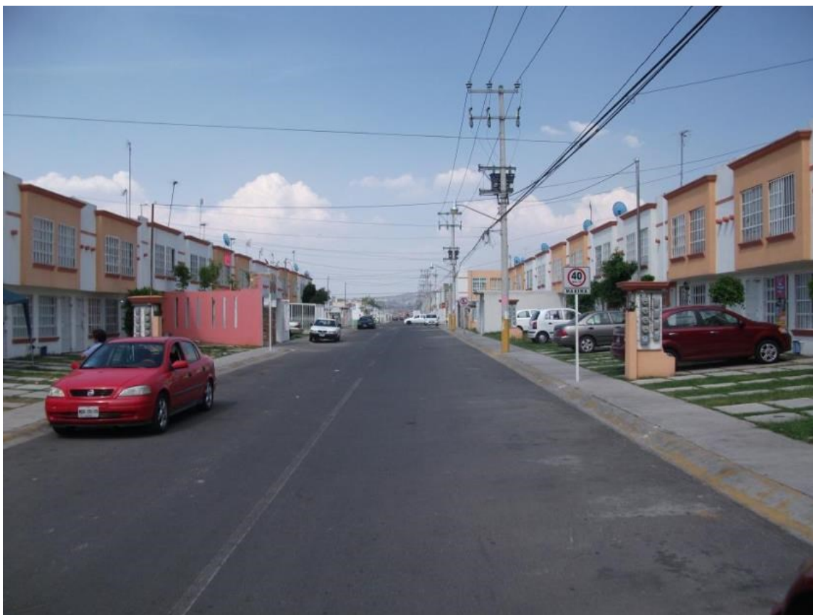
Figure 2.7 Commercially produced housing development, Los Héroes Ecatatepec (2012)
