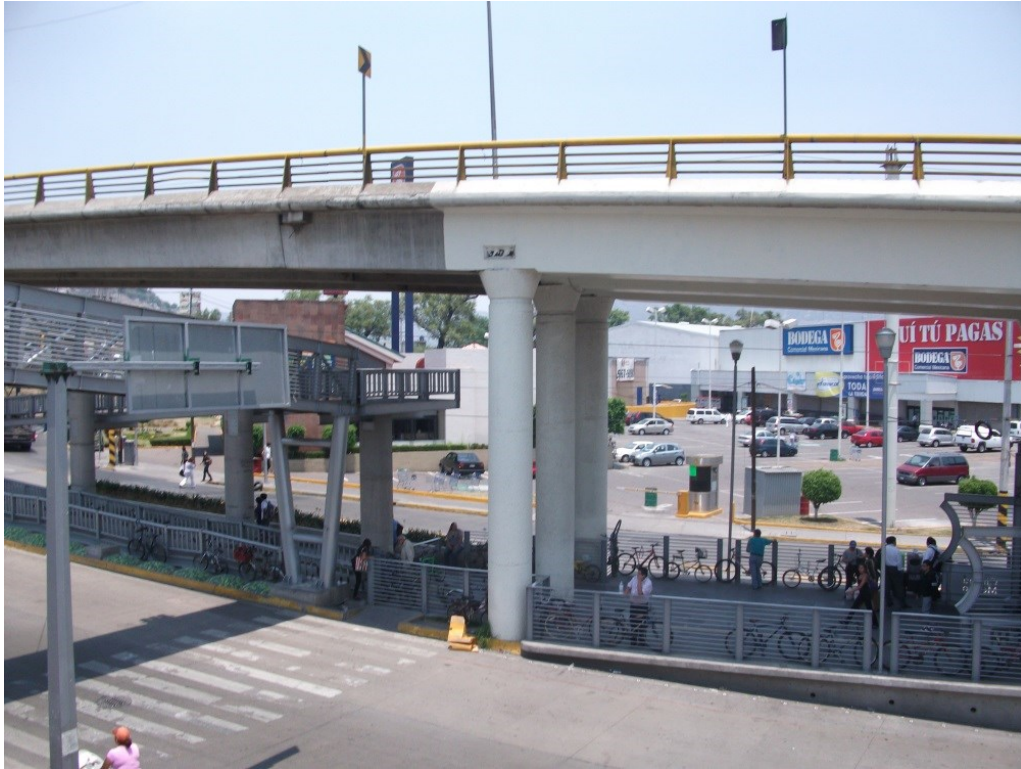
Figure 2.20 Pedestrian bridge crossing at Tenayuca Metrobus station (2012)
