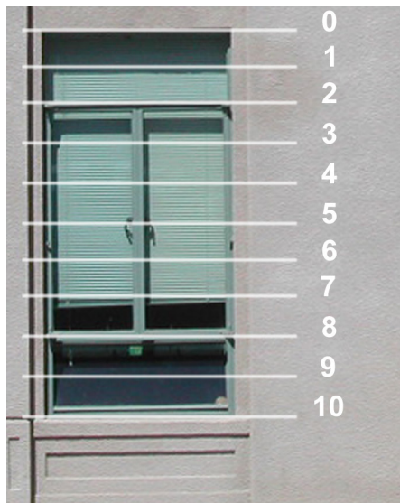
Figure 3.17 Window blind occlusion steps that were identified from time lapse photography (0 = fully opened, 10 = fully closed).
