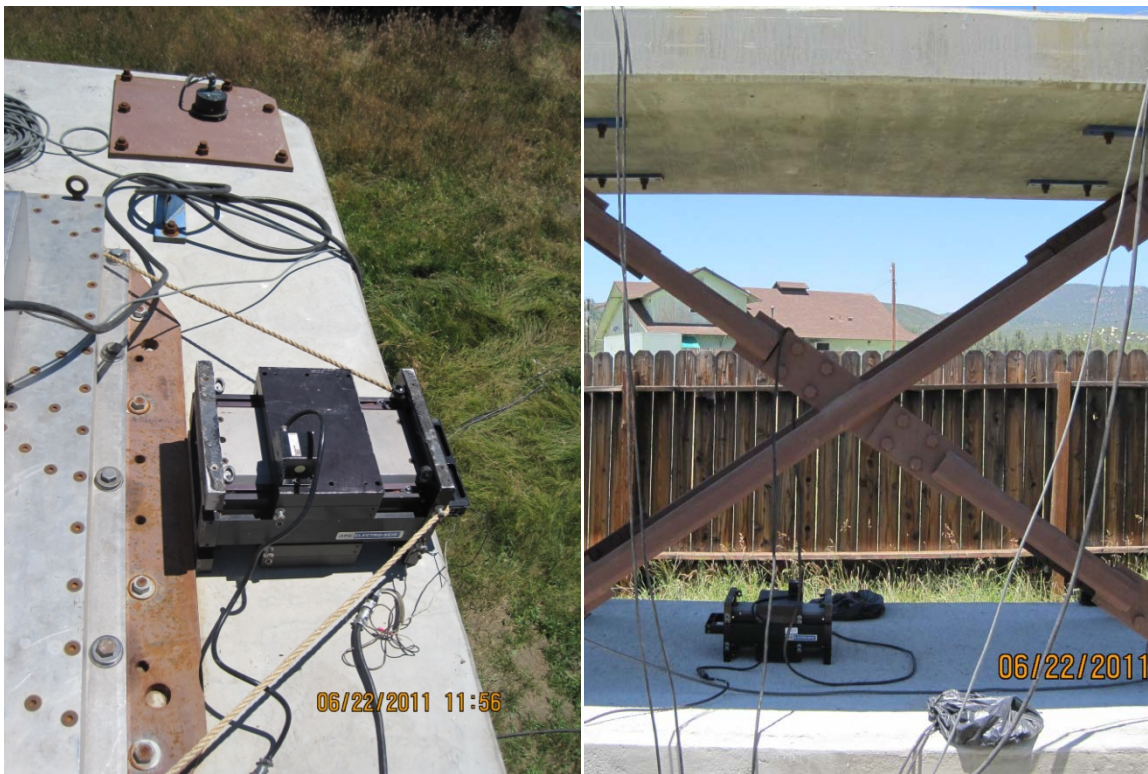
Figure 6-15 Photographs showing the Atom Ant shaker on the left, secured in-place with rope during forcing tests at the roof slab and on the right free-standing during forcing test at the foundation slab.
