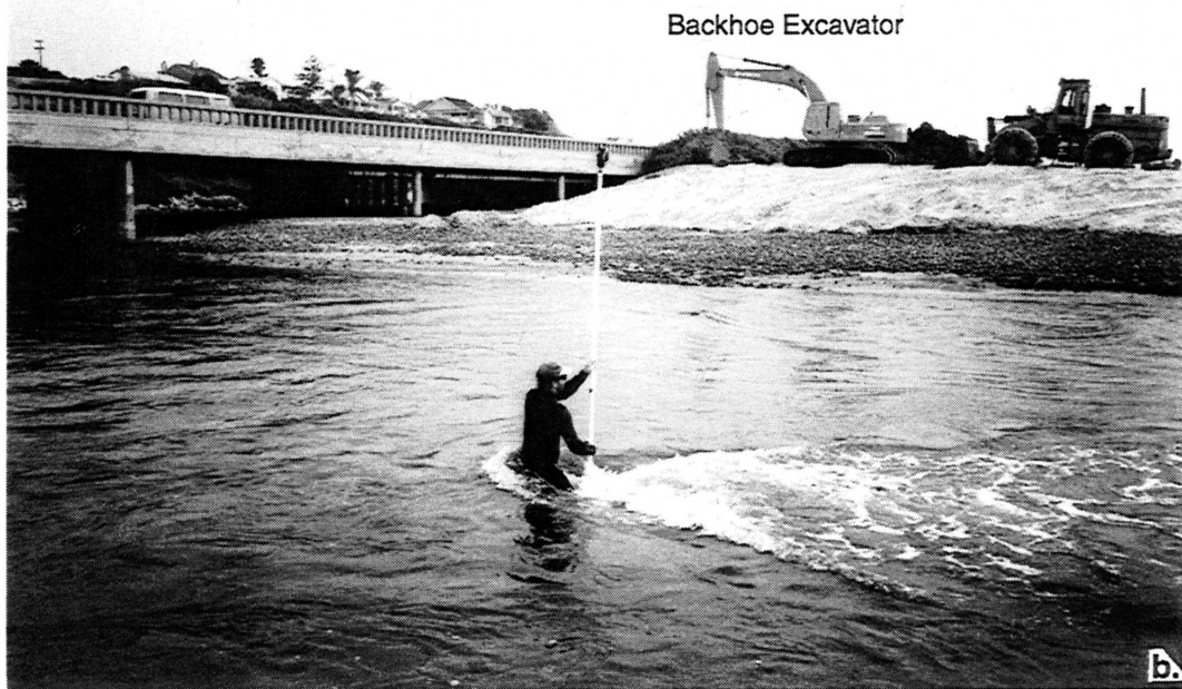
Figure 3. Conventional excavation equipment used to dredge San Elijo Lagoon.
